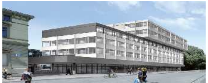
Stellwerk RailCity, Winterthur
